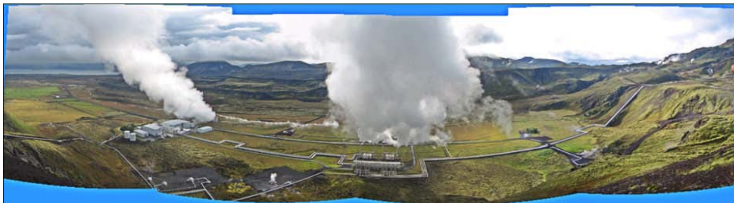
Active volcanism under the surface creates steam at the Nesjavellir power plant near Reykjavik. The geothermal power plant provides hot water and electricity to Iceland's major population center. (Photo credit: Tom Prettyman and Gil Esquerdo)
